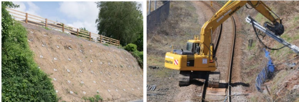
Figure 4-30 Typical Soil Anchor Installation
