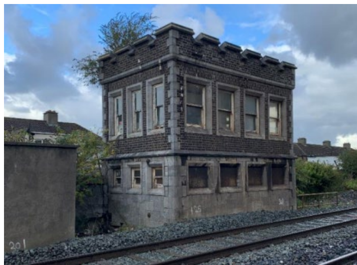
Figure 4-20 Old Signal Box - Inchicore Depot
